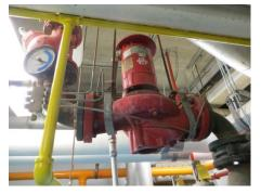
Primary Boiler Pumps Original to the building. Need replacing with energy efficient design.
